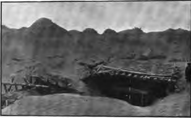
WOODEN GATEWAY OF RUINED QUADRANGLE, KARADONG, AFTER EXCAVATION.
