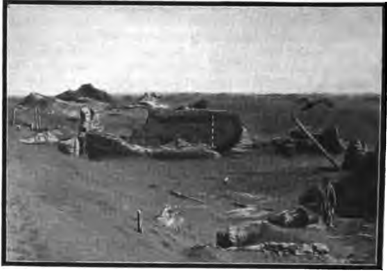
RUINED BUILDINGS WITHIN ENDERE FORT.
