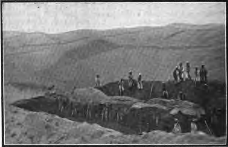
EXCAVATIONS PROCEEDING ALONG SOUTH-EAST WALL OF RAWAK STUPA COURT.
