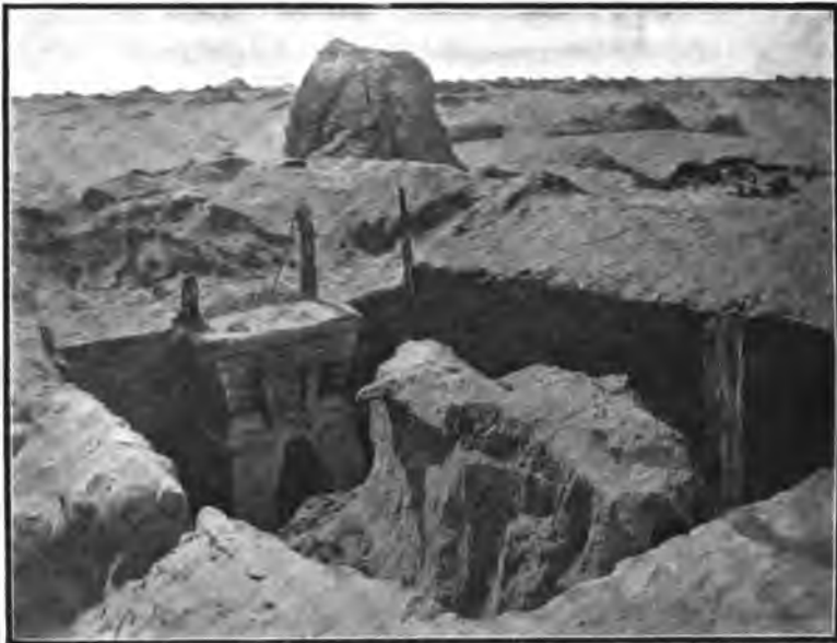
LOWER FLOOR ROOM OF RUINED DWELLING-PLACE, ENDERE FORT.
